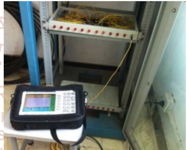
Figure 5: OTDR connected to fiber under test
