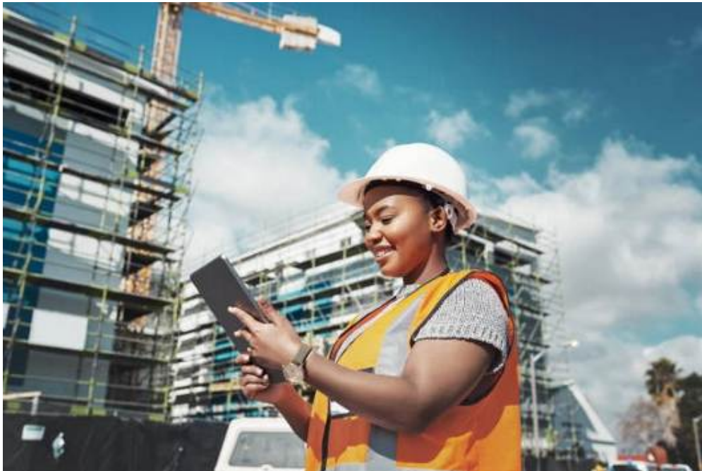
Figure 6 A construction site [13].
