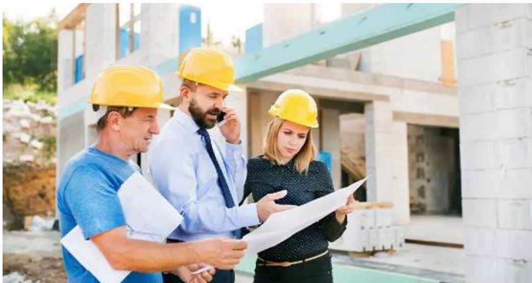
Figure 10 Some construction workers [15].
