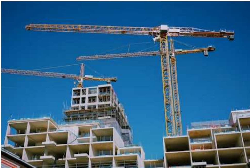
Figure 9 A construction site [14].
