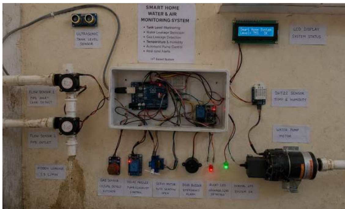
Fig. 1. Hardware prototype demonstrating integrated water leakage detection, tank level monitoring, and gas leakage detection with automated mitigation system.
