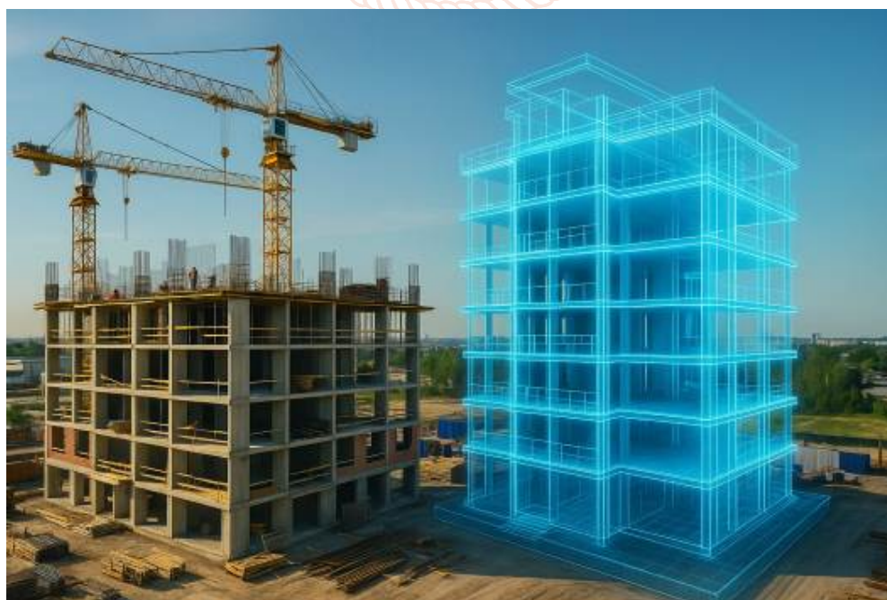
Figure 7 A building under construction [11].
