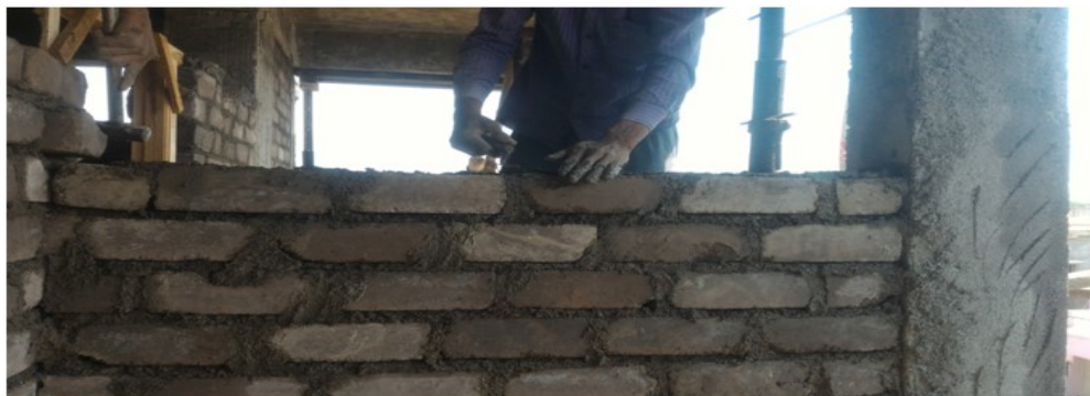
Fig4: E-bricks used in construction
