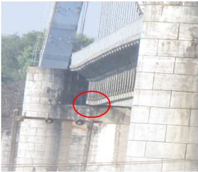
Fig. 5 Deflection of truss near Tower
