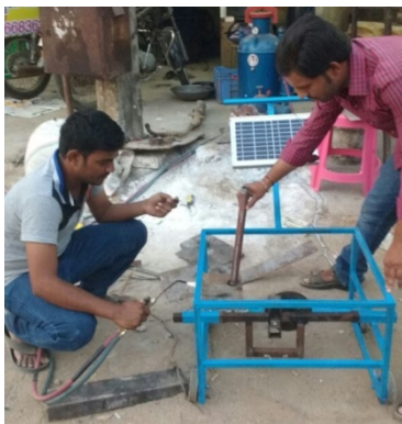
Fig. Mechanism frame welding
